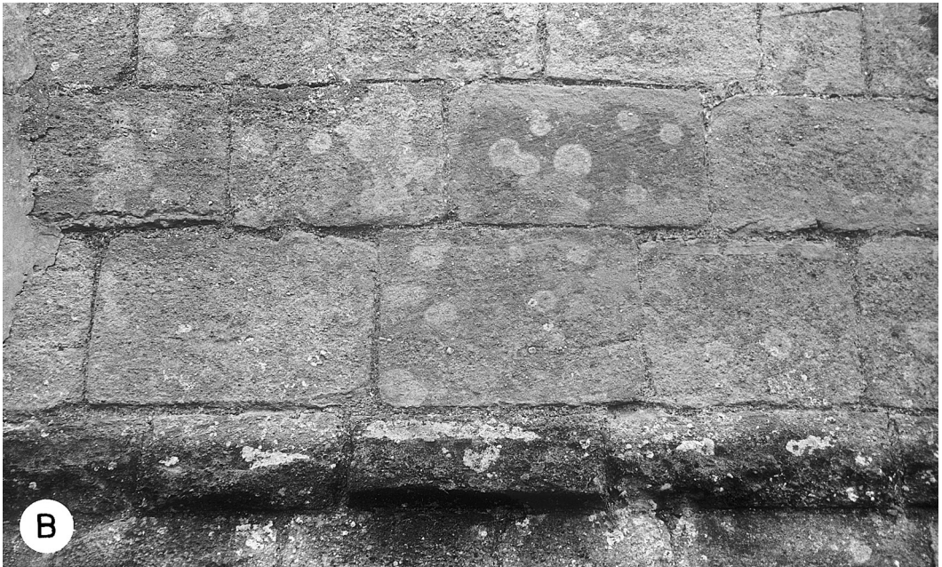
Fig. 7: Sudbrook Sandstone in castles. A – Plinth, south side, Great Tower, Chepstow Castle. B – Detail of ashlar and dripmould, Keep, Caldicot Castle.
