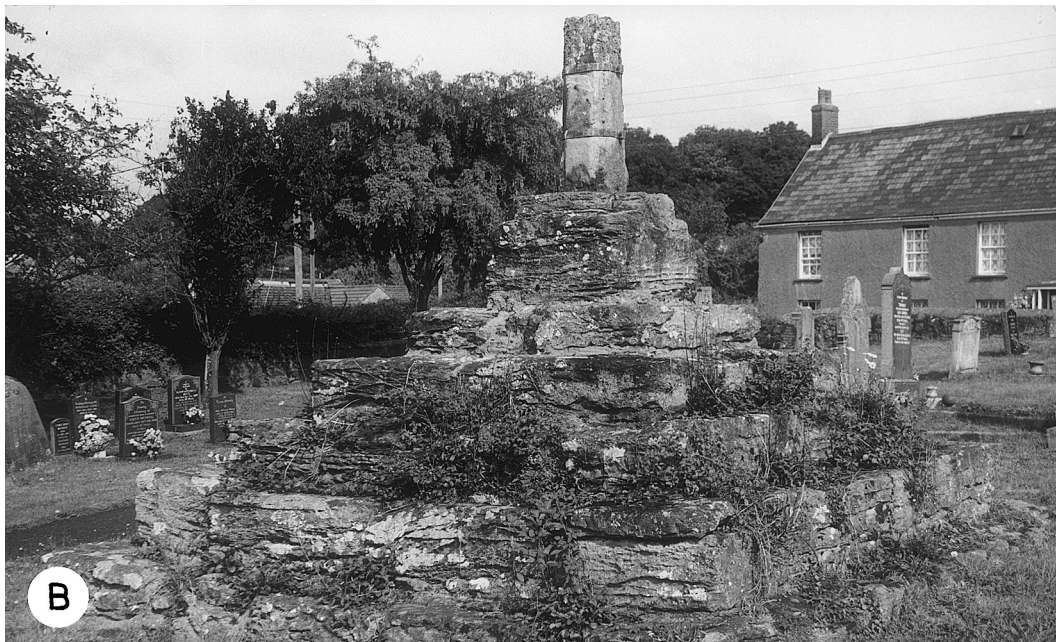
Fig. 6: Constructions in Sudbrook Sandstone. A – Detail of ashlar, St Mary’s Priory Church, Chepstow. B – Cross, St Mary’s churchyard, Portskewett.
