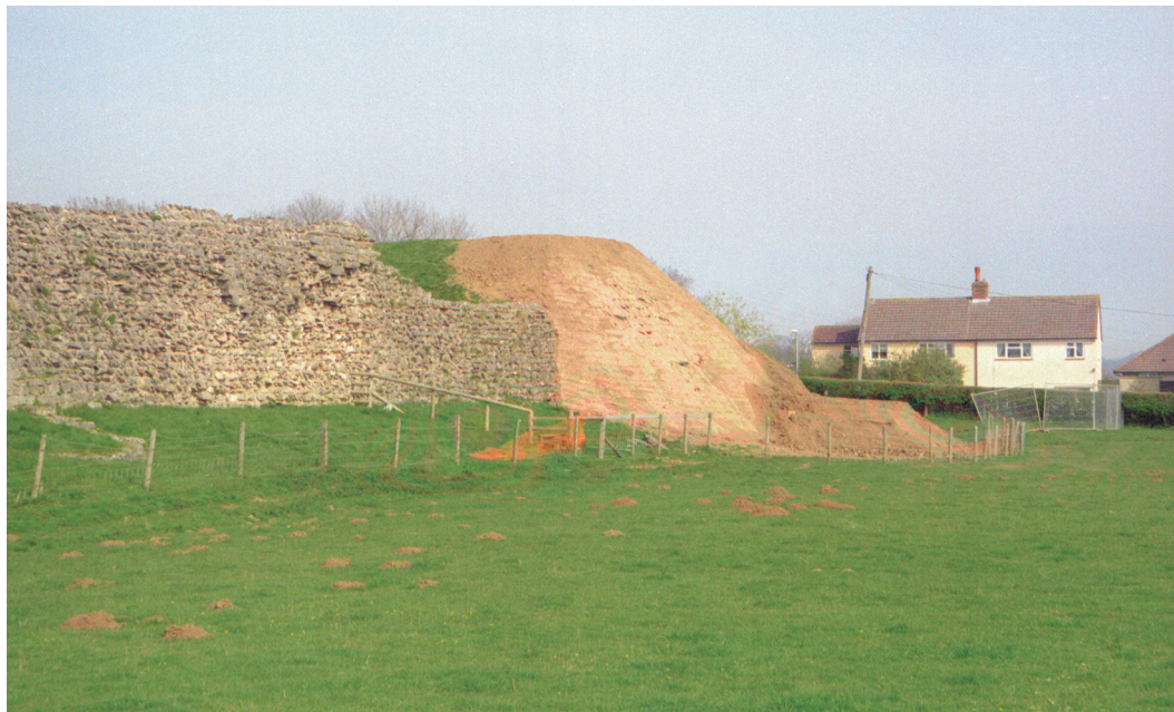
Plate 7: Caerwent motte . Reconstructed southern half (machine access ramp still in position). By courtesy of Cadw. Crown Copyright.
