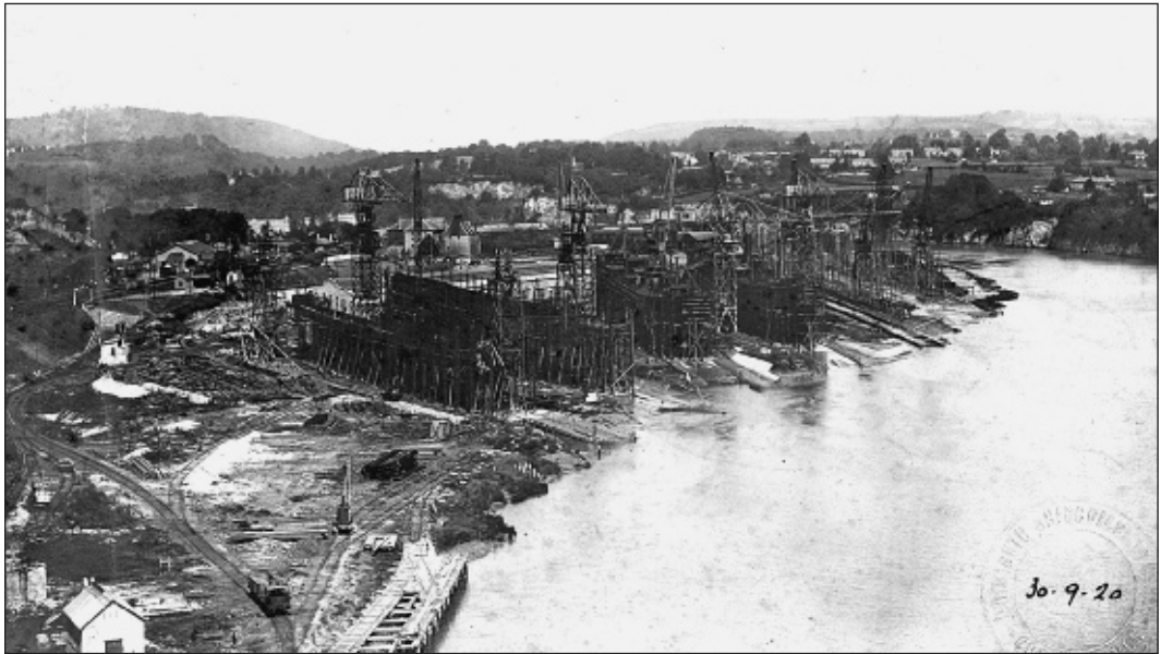
Fig. 33. 30 Sept. 1920. The day of the launch of War Odyssey from slipway No. 3, showing the War Genius , War Epic and War Idyll in increasing stages of completion. Note the stamp of the Monmouth Shipbuilding Company Ltd in the bottom right-hand corner. (Claire Field Collection).
