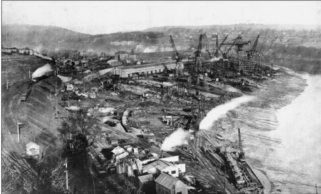
Fig. 31. Nov. 1919. Slipways Nos. 1 & 2 contain the War Glory and the War Iliad in the early stages of build, whilst scaffolding is being erected on slipway No. 3. (Claire Field Collection). Reproduced by kind permission of Mrs Claire Field.
