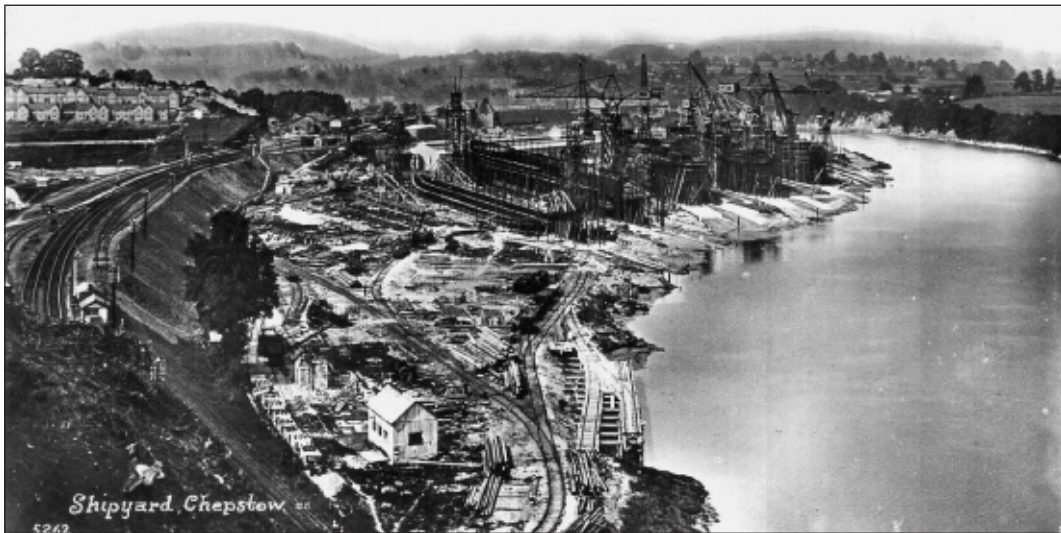
Fig. 32. May 1920. The War Glory had been launched from No. 1 slipway and the other five 'N' pattern ships were in various stages of completion with the War Idyll in slipway No. 6, just above keel height. (Claire Field Collection). Reproduced by kind permission of Mrs Claire Field.
