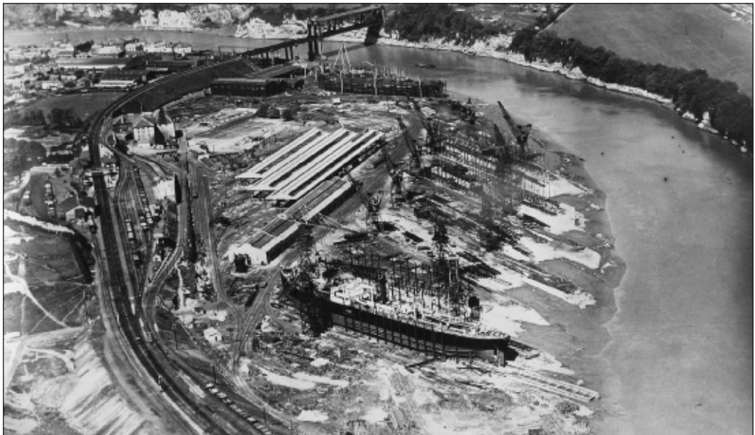
Fig. 34. Aug. 1921. The War Idyll ready for launching with the tanker Cynthia on the stocks in Finch's yard, near the bridge. Scaffolding has been taken down on slipways 5 & 4. (Claire Field Collection).
