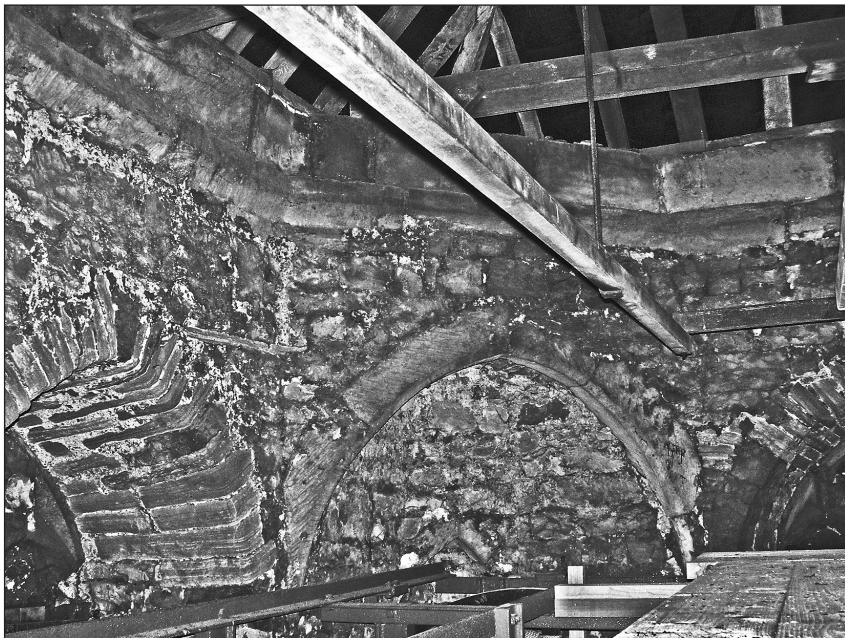
Fig. 11. The north-east tiered squinches of the tower of Caldicot parish church in 2008, looking north-east.
