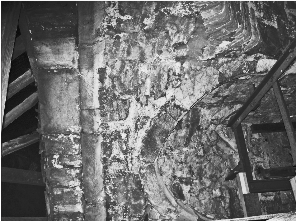
Fig. 12. Detail of the north-eastern tiered squinch of the belfry of the tower of Caldicot parish church in 2008.
