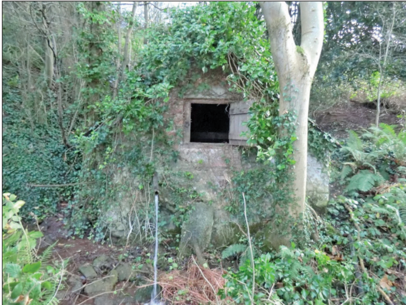
Fig. 12: West face of what may be Aram's second conduit house.
