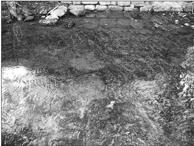
Plate 4.1: The bed of the Dowlais showing paving slabs laid in the stream bed. Photograph: D. Standing.
