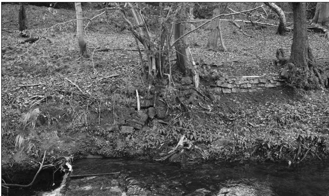
Plate 7: Site 11 – The south bank. Providing evidence for the Dowlais Brook being walled along its possible outer precinct boundary. Photograph: D. Standing.
