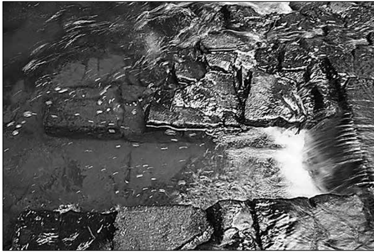
Plate 3.2: The outlet for the lower sluice gate at site 9. Photograph: D. Standing.
