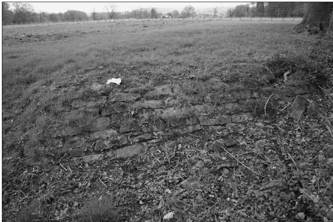
Plate 5: The stone lining of the fishpond that adjoins site 11. The masonry lines up with the evidence for the rebuilt dam structure within the north bank of the Dowlais. Photograph: D. Standing.
