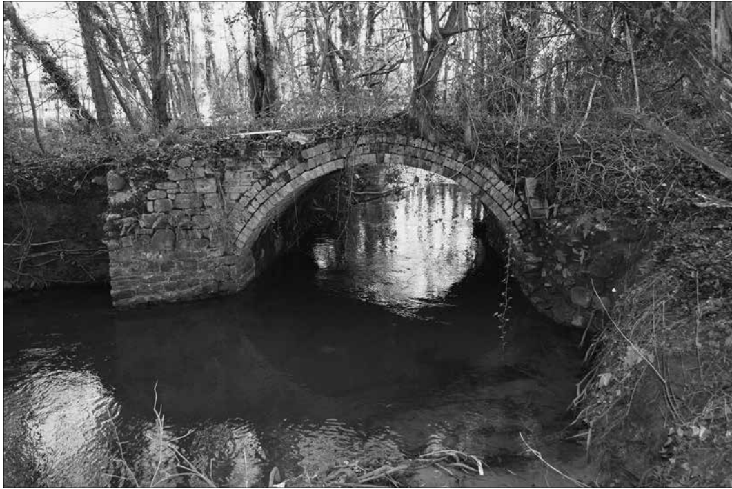
Plate 2: The bridge located at site 4 is 4.2m wide and 2m high. Probably rebuilt in the 19th century, the architectural and geomorphological evidence indicate the Dowlais Brook had a much greater width at the time of its construction. Photograph: D. Standing.
