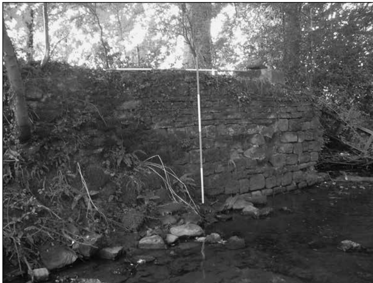
Plate 4: Looking downstream at the northern bank remains of the fishpond dam. Just above the 1m high mark, there is evidence for the dam being rebuilt during the post medieval period. The archaeology remaining within both banks and across the Dowlais is considerable. Photograph: D. Standing.
