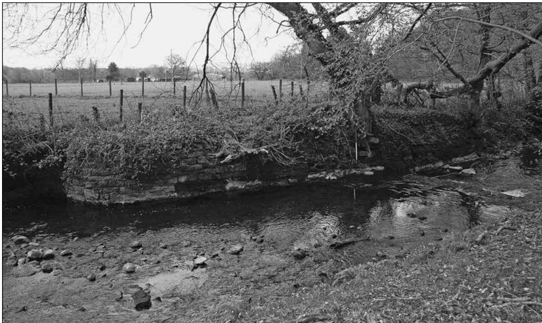
Plate 6: Site 11 – The north bank. The masonry curves out of the perpendicular into the bank. At over 20m long, they appear to be complete. Photograph: D. Standing.
