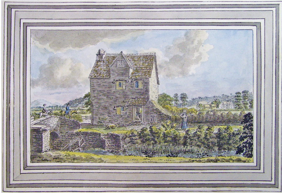
Fig. 7: 'Bridge over the Pelth brook, with a distant view of Readymain. J.G. 1805'.
