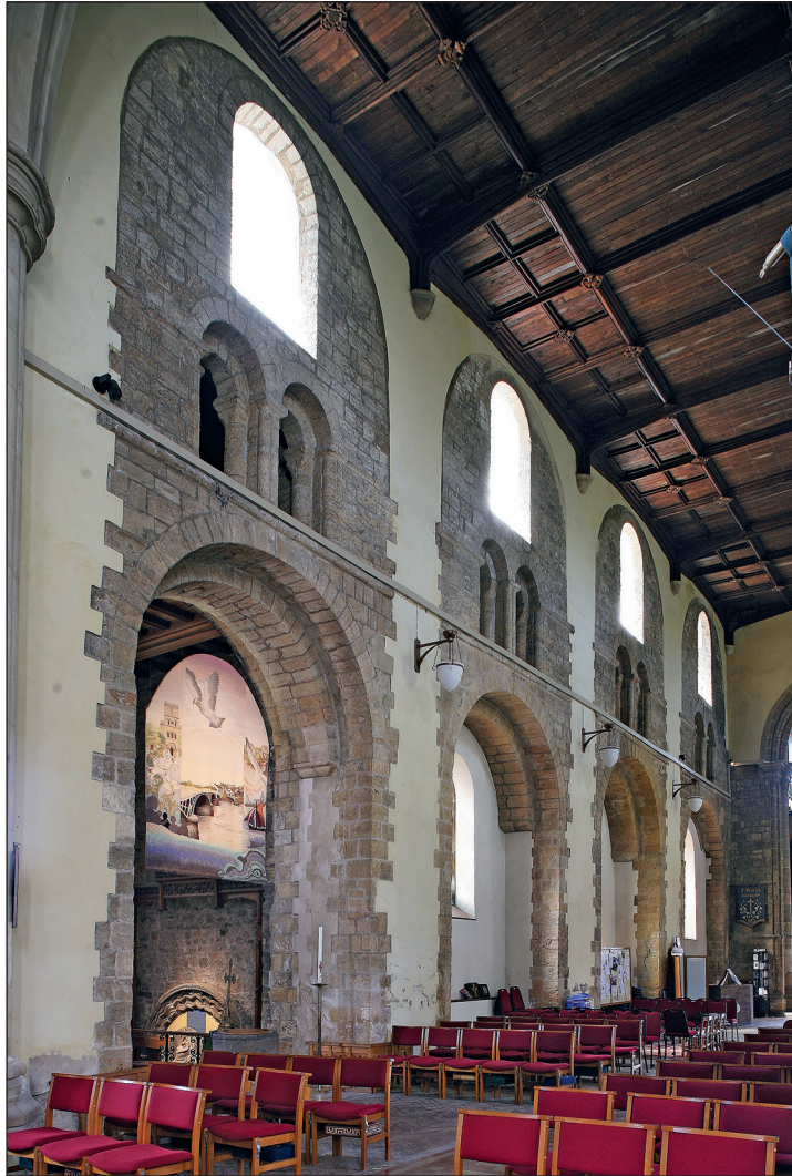
Fig. 3. Chepstow Priory, nave interior, S elevation.
